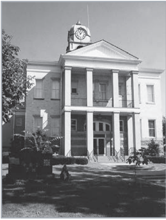
Adams County Courthouse West Union
