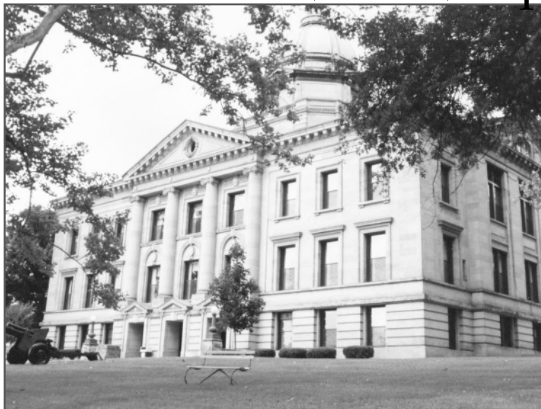
Lawrence County Courthouse Ironton
